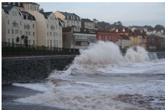
Figure 1: Wave overtopping along the Dawlish frontage
