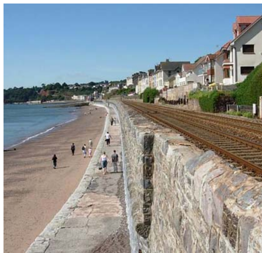
Figure 2: King Harry's Walk, north of Dawlish Station
